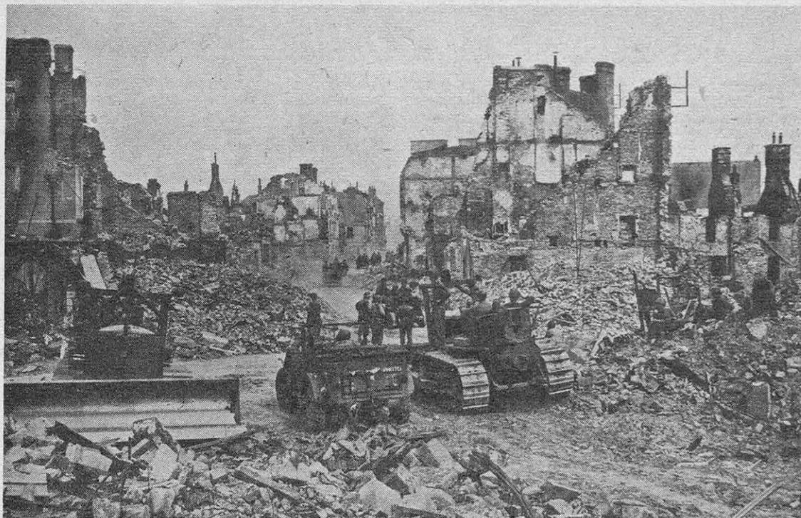
FIG. 9. — LES BULLDOZERS ONT FRAYÉ UN PASSAGE A TRAVERS LES DÉCOMBRES DE SAINT-LO (U. S. INF. S.)
