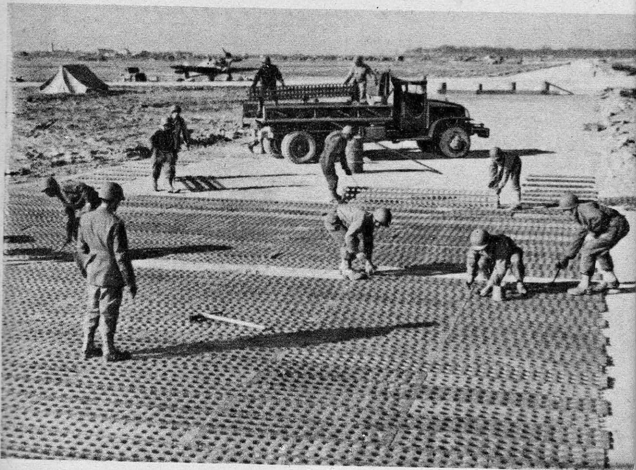
FIG. 8. — LA CONSTRUCTION D'UNE PISTE D'ENVOI EN TOLES PERFORÉES
