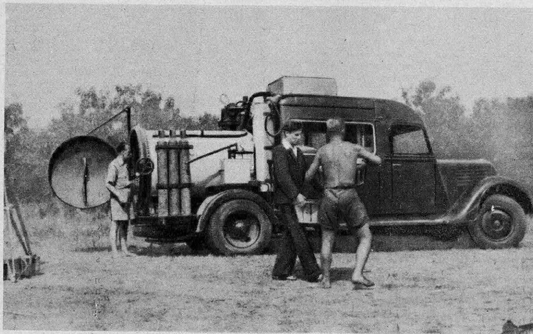
FIG. 1. — CAMION AUTOCLAVE SERVANT A TRAITER LES FRUITS PROVENANT DE VERGERS PARASITÉS AVANT LEUR EXPÉDITION, PRÉCAUTION INDISPENSABLE POUR ÉVITER LA DIFFUSION DES PARASITES
