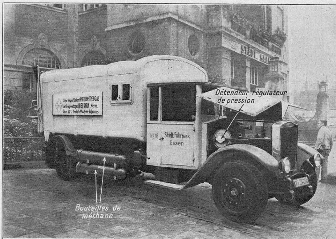
FIG. 3. — EN ALLEMAGNE, PLUSIEURS CENTAINES DE VÉHICULES UTILISENT MAINTENANT COMME CARBURANT LE MÉTHANE MIS EN BOUTEILLES SOUS HAUTE PRESSION
