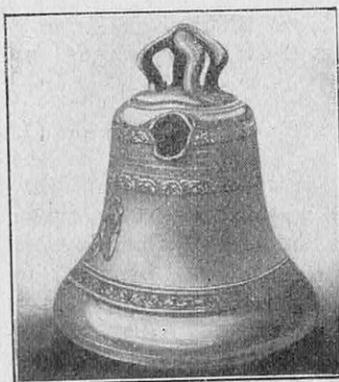
FIG. 1. — LA FUSION DE CETTE CLOCHE, FRAPPÉE PAR LA FOUDRE, EST UNE PREUVE DE LA GRANDE INTENSITÉ DE COURANT QUI CIRCULE DANS L'ÉCLAIR
