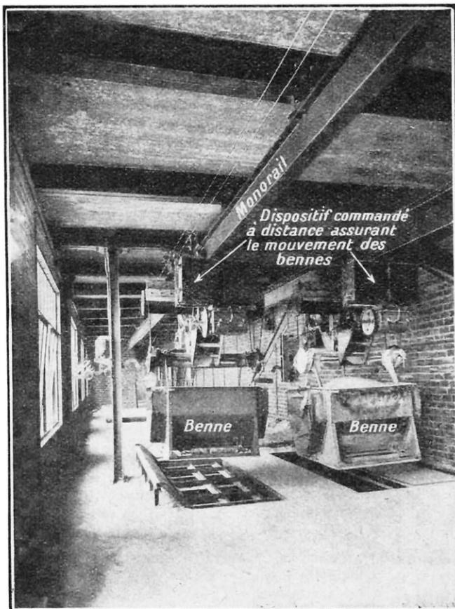
FIG. 5. — VOICI DES BENNES, UTILISÉES POUR LE TRANSPORT DE PRODUITS CHIMIQUES, DONT LES MANŒUVRES SONT COMMANDÉES A DISTANCE
